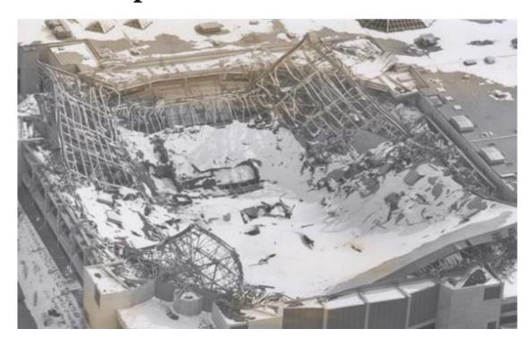
In January 2006, "the roof of one of the buildings at Katowice International Fair collapsed in Chorzów / Katowice, Poland." Subsequently, "a forensic investigation found numerous design and construction flaws that contributed to the speed of the collapse. The snow from the roof was not being removed which resulted in construction overload by more than 100%."
